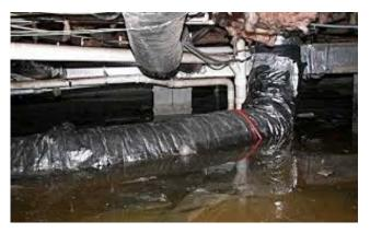
Moisture: Excessive condensation was found in the crawl space. This condensation can cause wood rot and the growth of fungus that can destroy wood. The crawl space should be thoroughly dried by a qualified moisture control specialist. The crawl space poses a safety concern.
